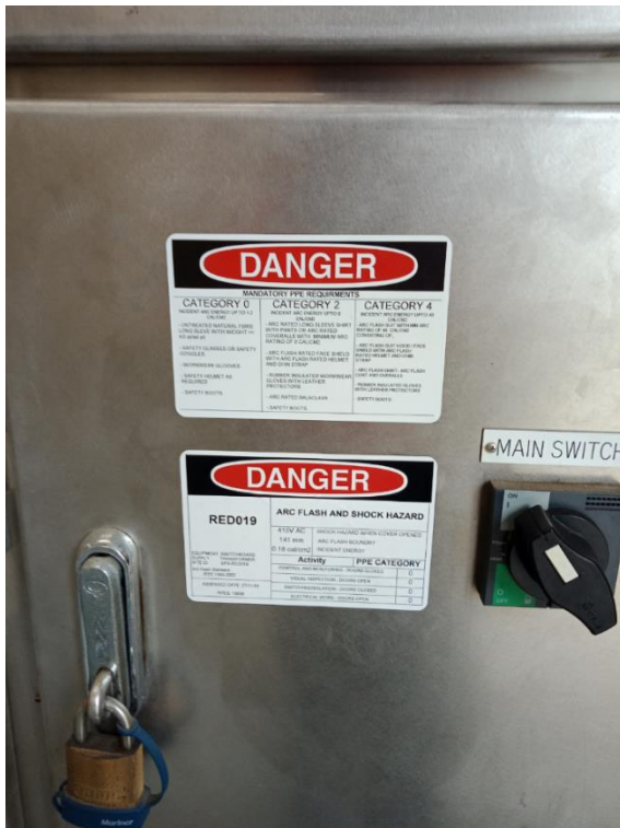
*Additional Type 3 label is required on BUS/Load side if Cat2 or above PPE when running on generator
