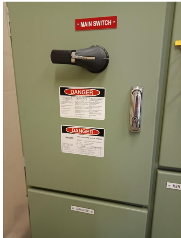
*Additional Type 3 label is required on BUS/Load side if Cat2 or above PPE when running on generator
