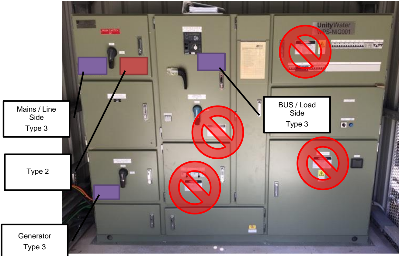
*Additional Type 3 label is required on BUS/Load side if Cat2 or above PPE when running on generator
